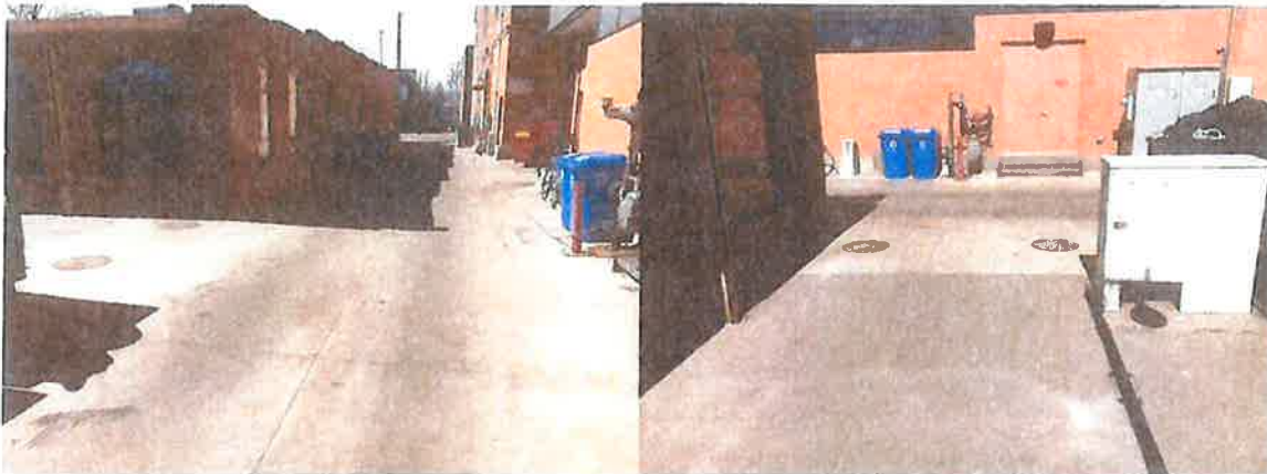
Grease Vault Covers (looking west)
